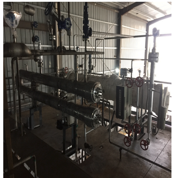
(b) On-site installation of the superheater
